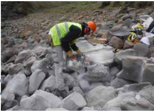
6. Trimming sandstone overburden to free the boulder.
